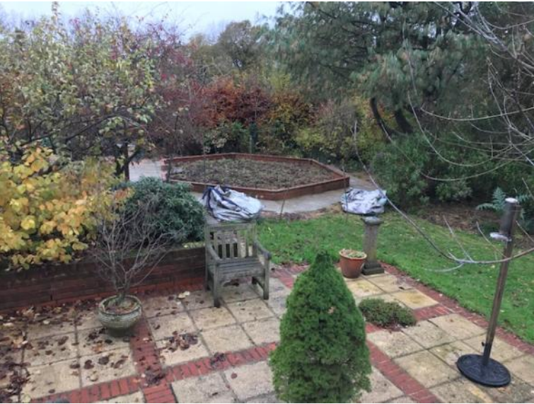
... Autumn 2019 - brick foundations and path completed
