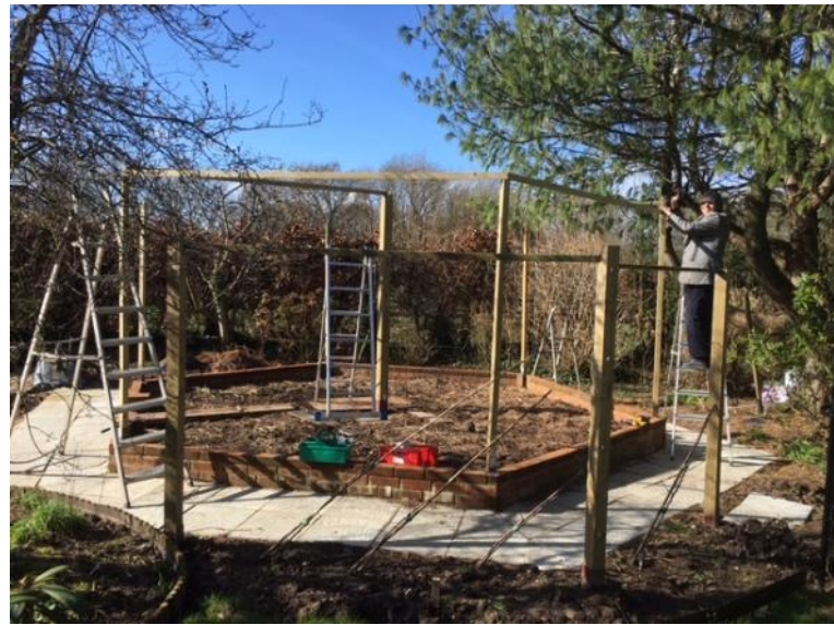
February 2020 - wooden framework almost completed ...
