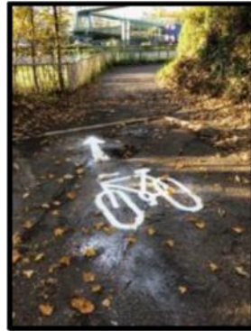
A new, wider cycle and pedestrian pathway with dropped kerb at the southern end of The Street to access the A27 flyover
